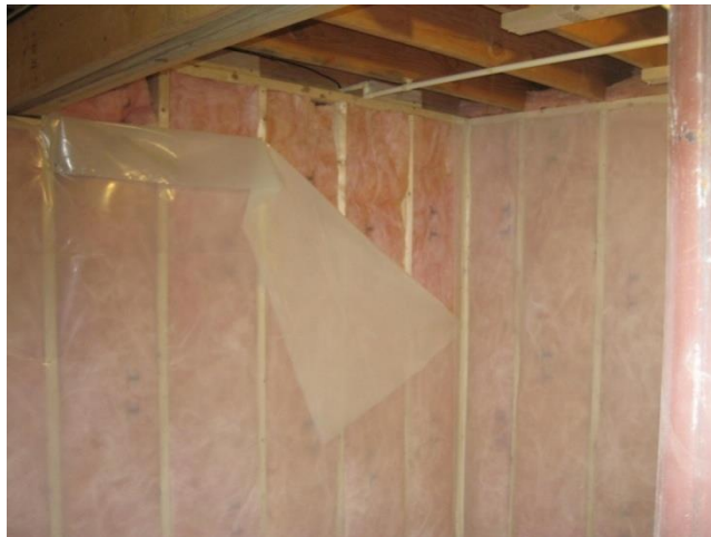
Figure 27: Grade II Fiberglass Batts—Basement Walls in Newly Constructed Home
