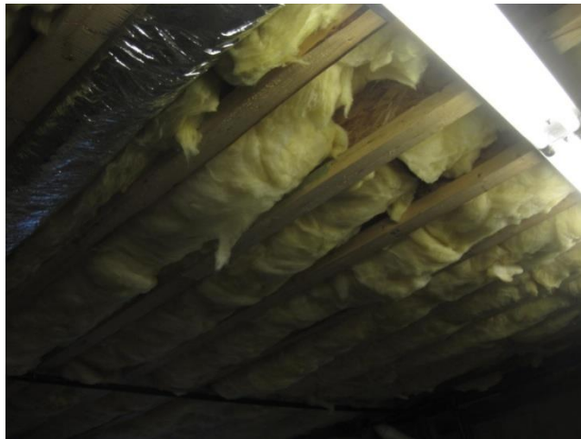
Figure 30: Grade III Fiberglass Batts—Frame Floor in Newly Constructed Home
