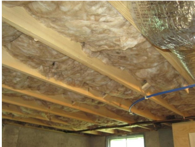
Figure 29: Grade II Fiberglass Batts—Frame Floor in Newly Constructed Home
