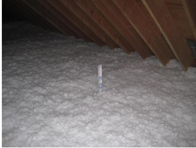
Figure 31: Grade I Blown Fiberglass—Attic in Newly Constructed Home
