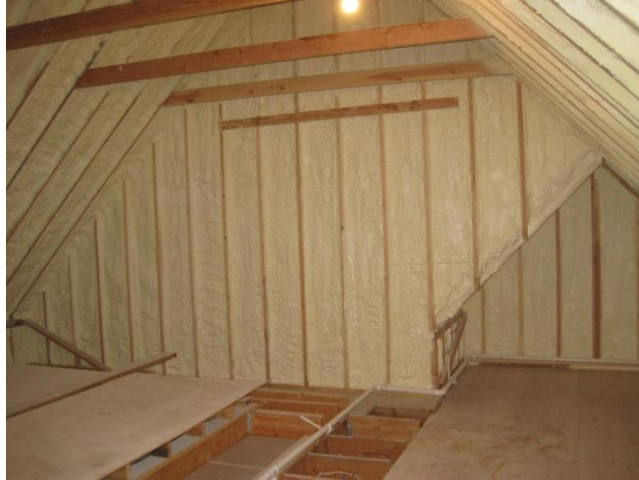
Figure 26: Grade I Closed Cell Spray Foam—Exterior Walls in Newly Constructed Home
