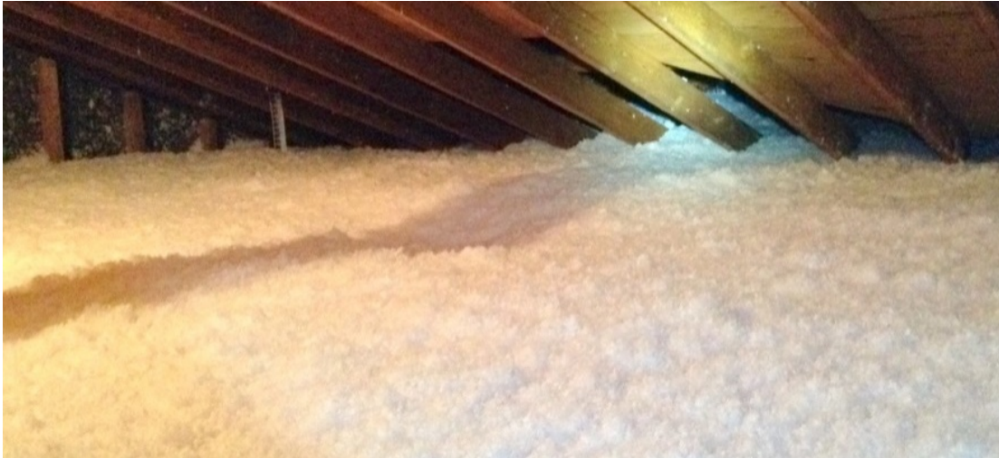
Figure 5: High Quality Blown-in Attic Insulation
