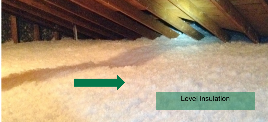
Figure 20: High Quality Blown-in Attic Insulation
