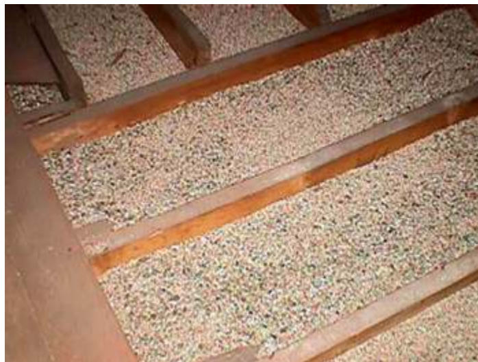
Figure 4-4: Vermiculite Insulation between Attic Rafters
